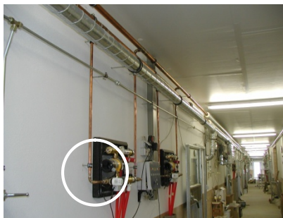
Illustration 14: Wrong - insulation lacking in the entire piping system
