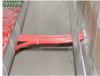
Illustration 13: Supply pipes in the channel
