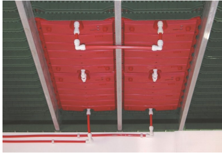
Illustration 12: Connecting the Thermo W with the push-fit connection system
