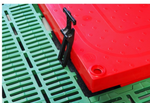
4. use tool as pedestal holding up the panel
